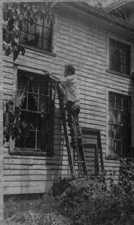
JAMES DOMINICK scrapes away at the countless layers of paint covering the siding. He only takes a day or two of his vacation at a time to keep the work from becoming boring.
